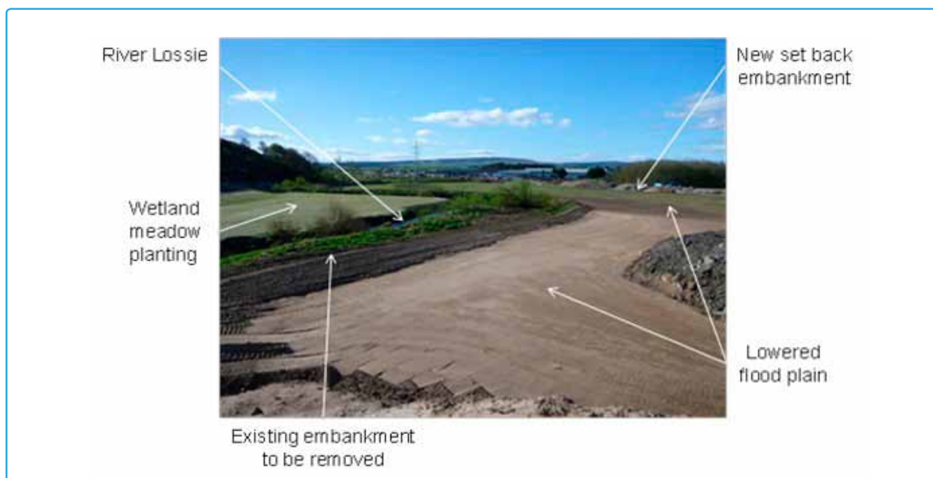
New flood alleviation measures at Elgin after construction
